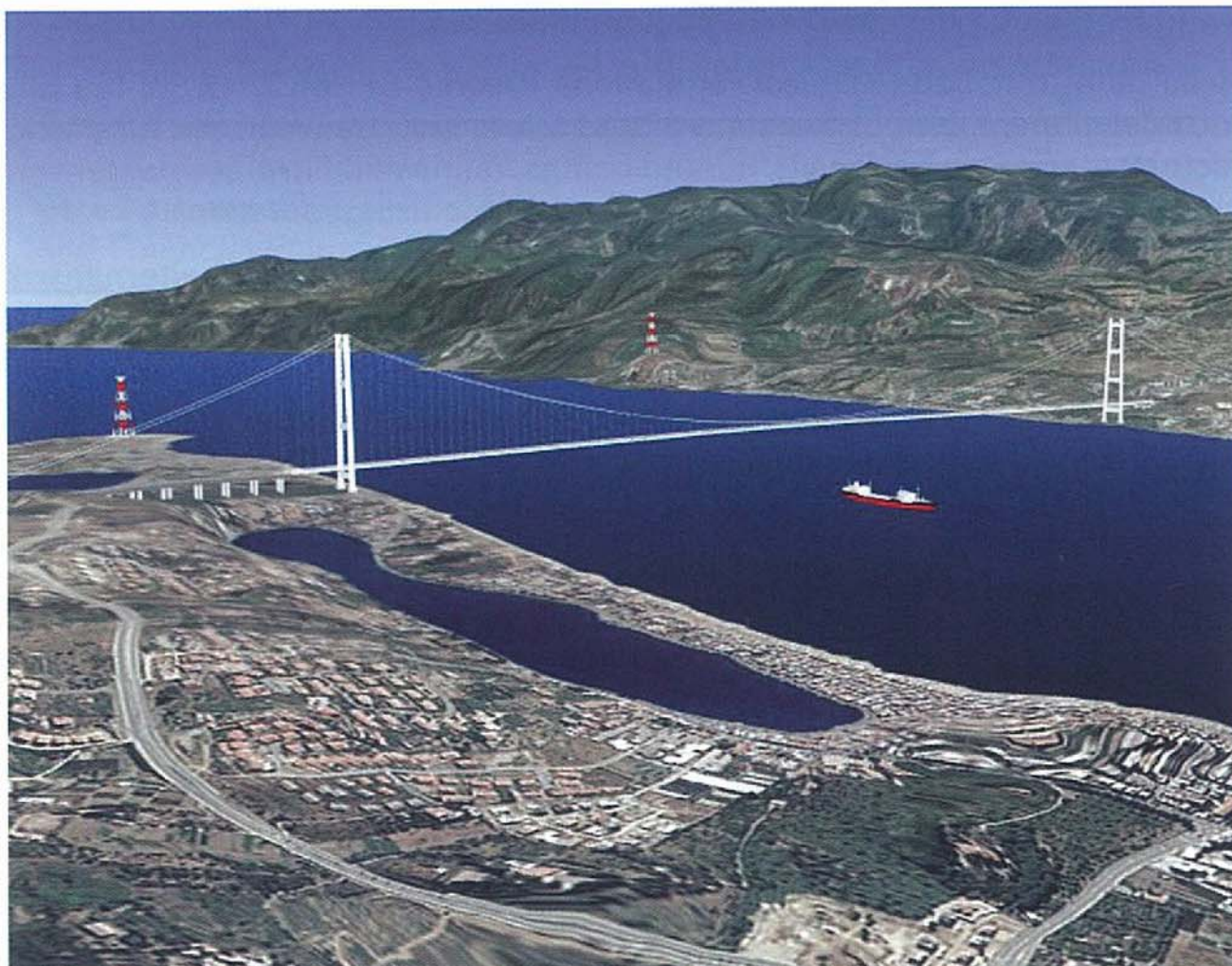
Figure 3.5 ► Visual impact assessment by 3D interactive modelling: view of the bridge from Sicily.
